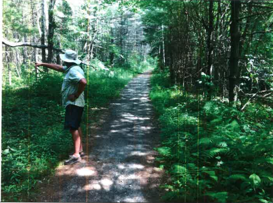
Photo 17. Conservation Commission Vice Chair Jon Clements examines the trail on a recent walk-through. The right-of-way here would safely accommodate a 10-foot wide travel surface and a 2-foot grassy shoulder on each side. There might also be room for a parallel horse trail at one side.
