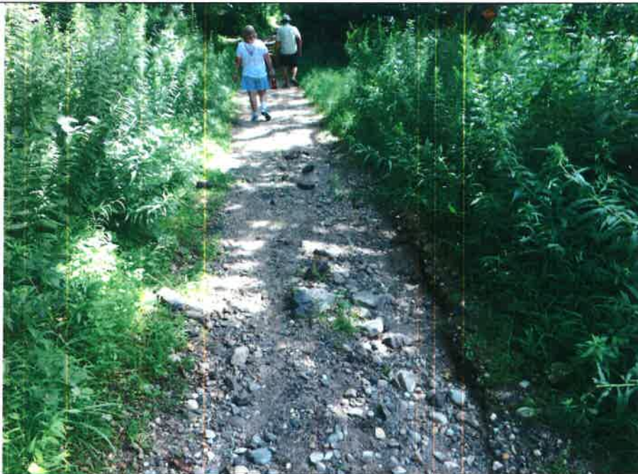
Photo 2. Looking southeast from Springfield Road at the beginning of the route. Road runoff has eroded some of the surface of the trail in this section. The right-of-way here would accommodate a 10-foot wide travel surface plus two 2-foot grassed berms at either side.
