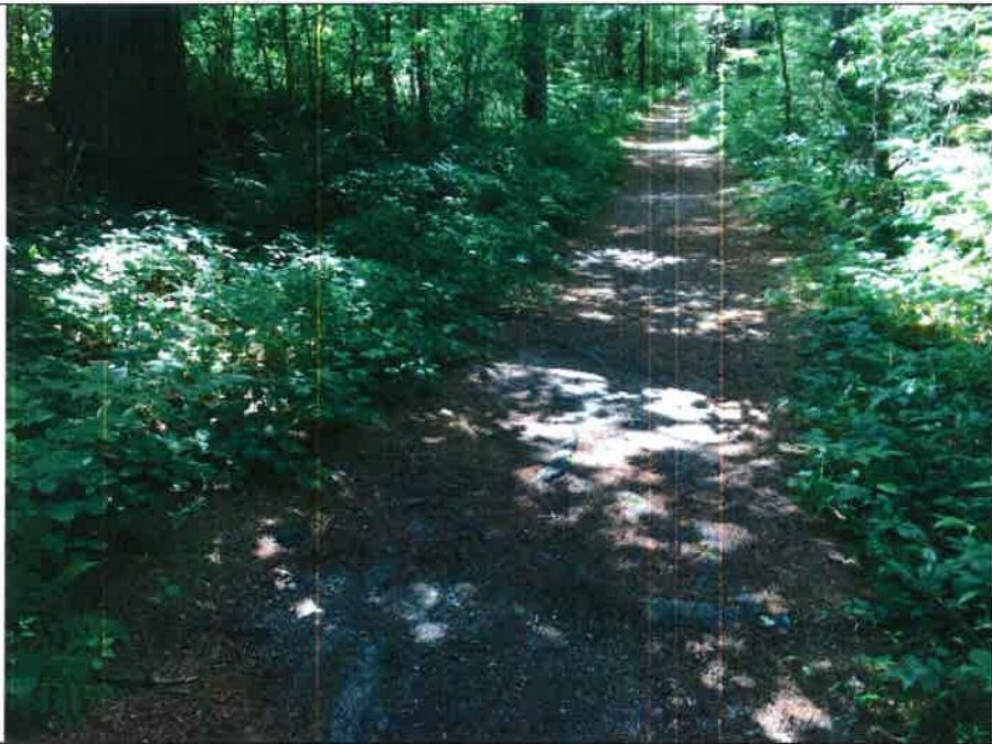
Photo 7. Tree roots that are raised above the present travel surface would have to be removed to allow installation of a gravel base and provide a stable trail bed. This section is a short distance northwest of the North Washington Street crossing.
